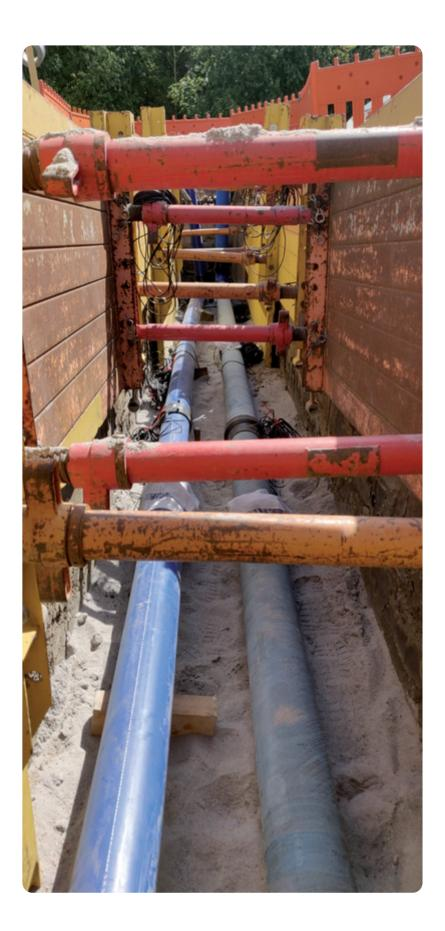
Construction of a trench with two drinking-water supply pipes made of cast iron and polyethylene, respectively. Photo courtesy of Claus Haslauer, VEGAS, University of Stuttgart, Germany.
